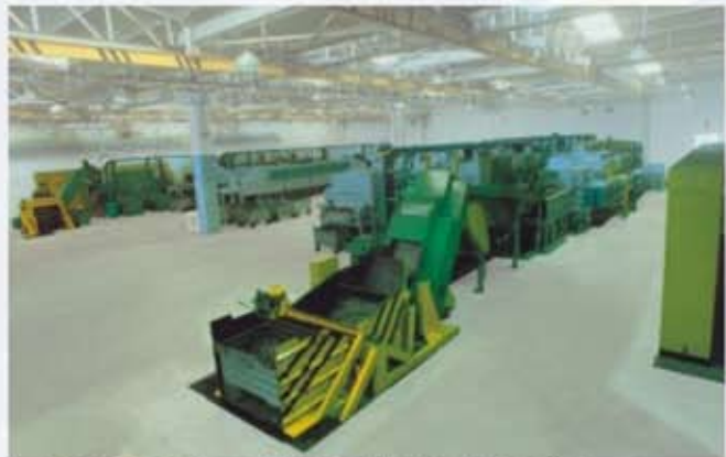
Two 'Bin to Bin' Continuous Hardening Plants for Bearing Rings
