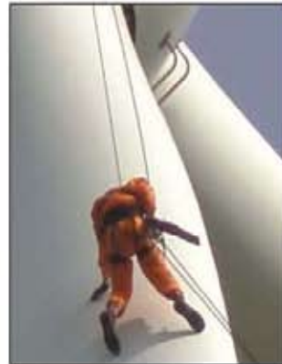
Blade Inspection using Rope Access
